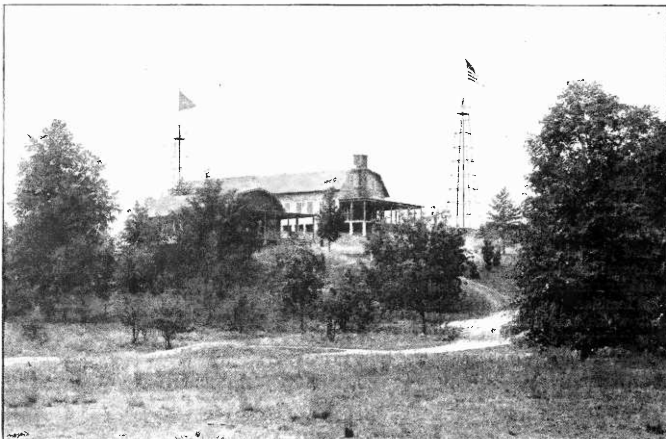
THE WIRELESS TOWERS AND RECREATION BUILDING AT CAMP WALLKILL, NEAR LAKE MOHAWK, N. Y.
